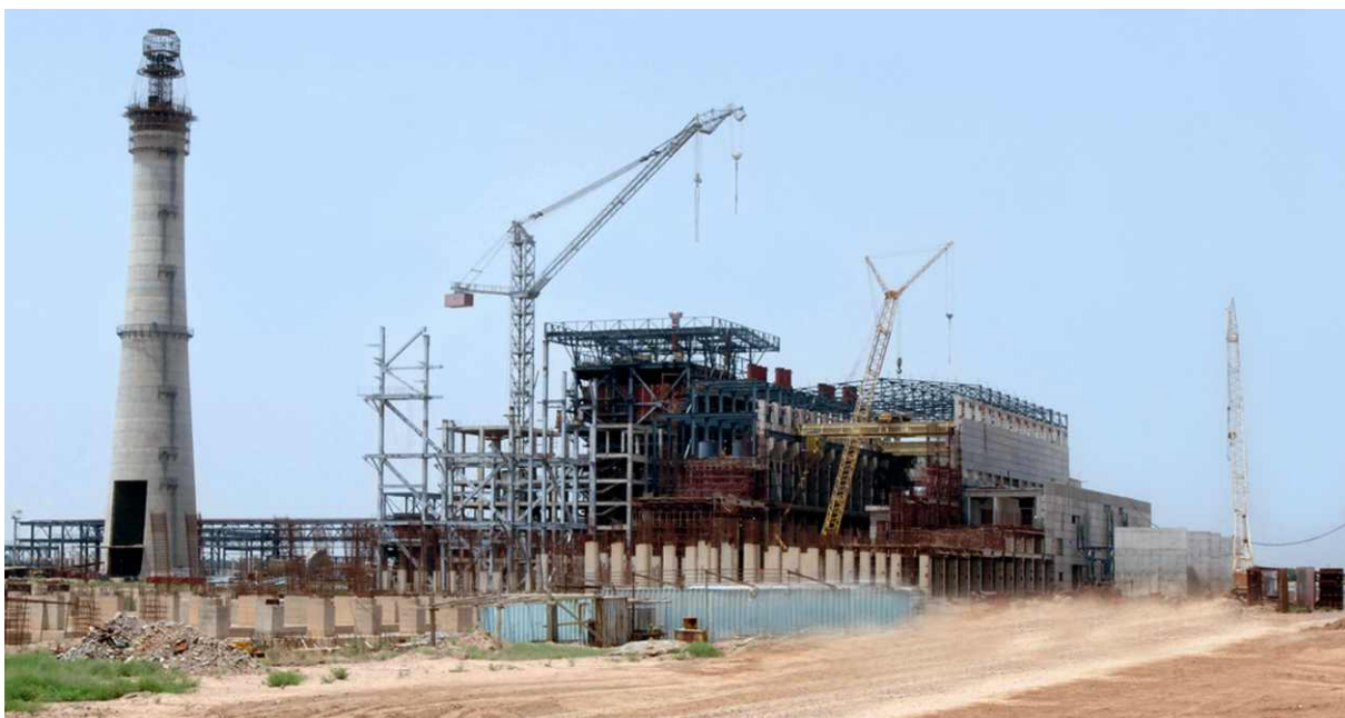
Rehabilitation of a power station
